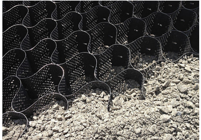
Figure 9. Geocells partly filled with aggregate
