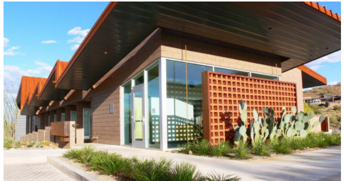
FIGURE 21—Concrete Masonry Screen Walls
