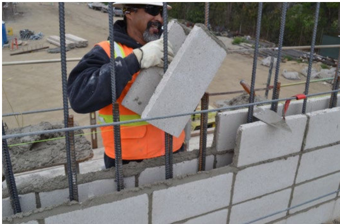
FIGURE 6—Installation of Open-End Units
