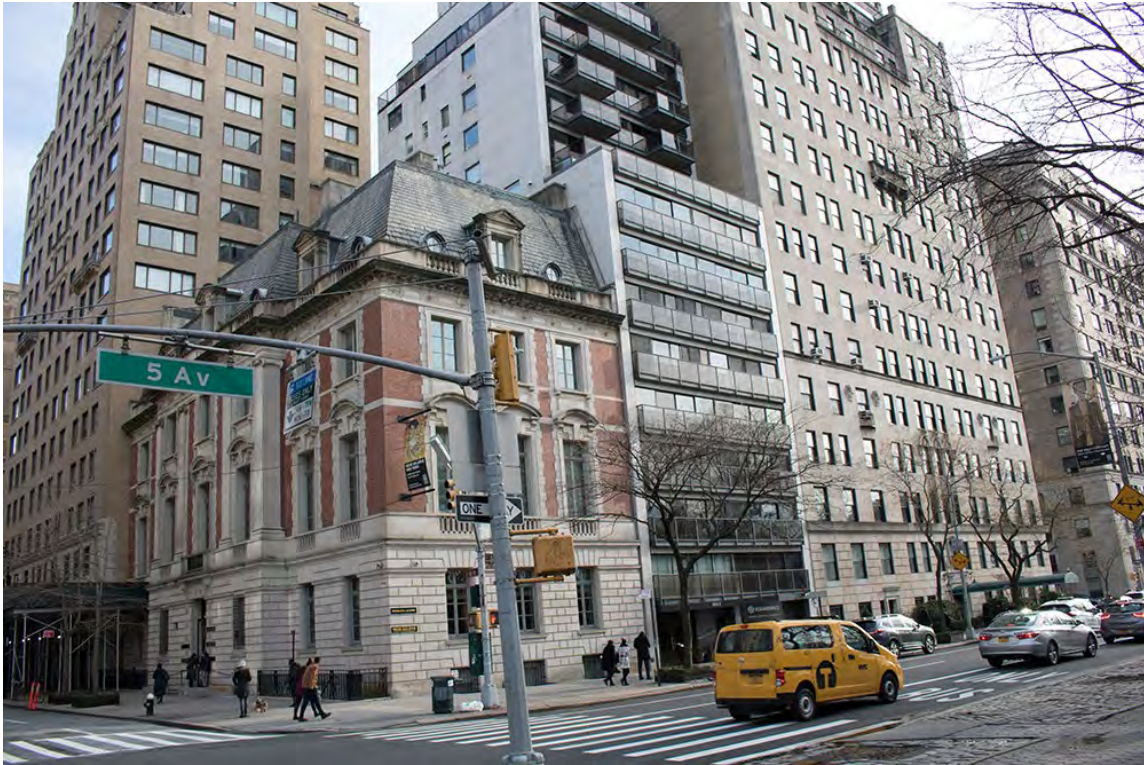
Project Site, Neue Galerie, 5 th Avenue and E. 86 th Street
